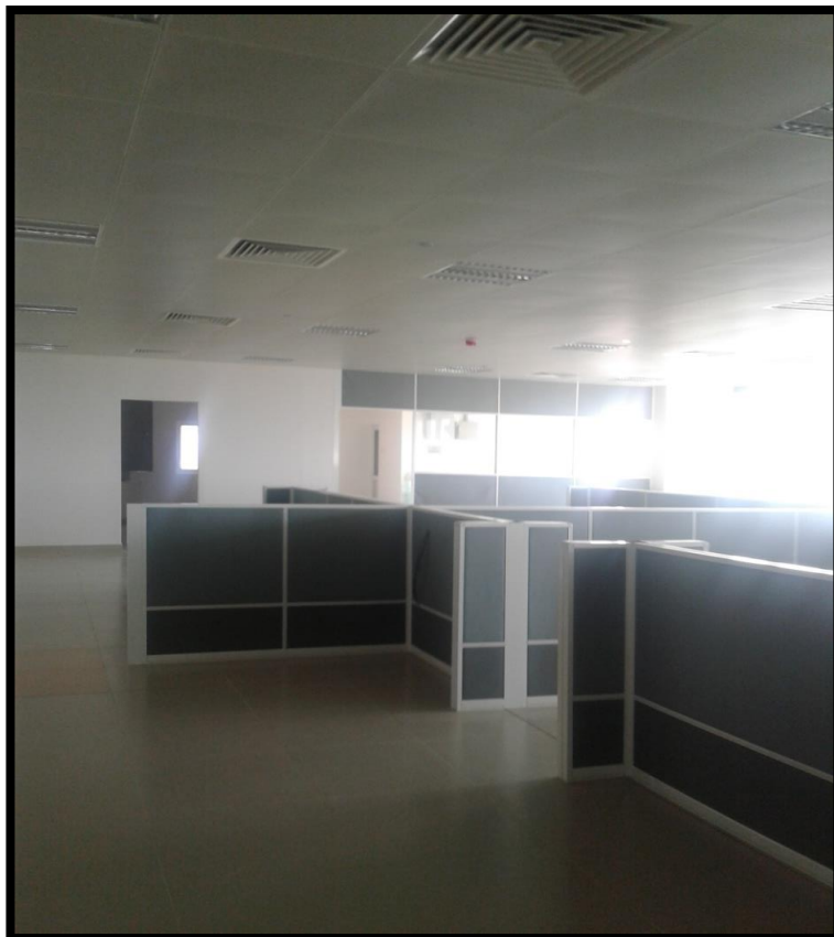
8 th Floor Complete Partition Work
