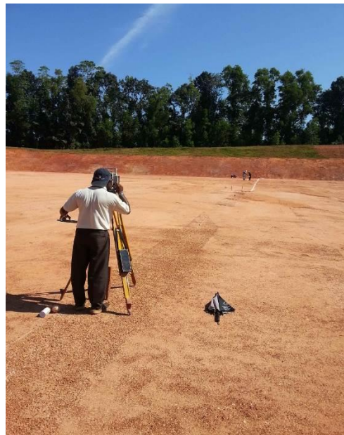
Demarcation of point height and center line
