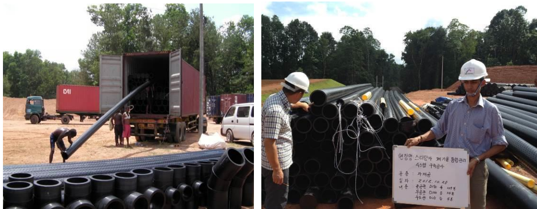
Drainage & Leachate collection tubes
