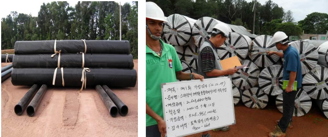
Landfill liners being carefully stored at the site
