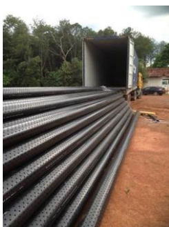
Unloading of Drainage and Leachate piping at the site, Dompe
