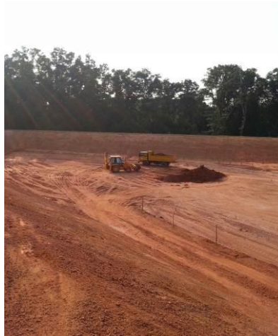
Removing of top soil
