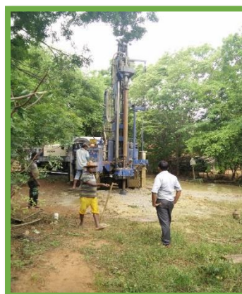
Tube well drilling under kirindi oya project
