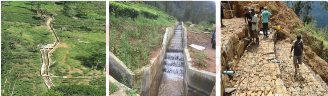
Garandiella Landslide Mitigation Project work in progress
