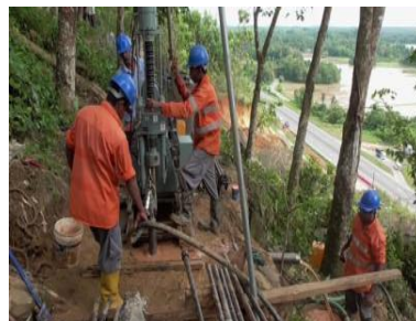
Geotechnical Investigation in progress
