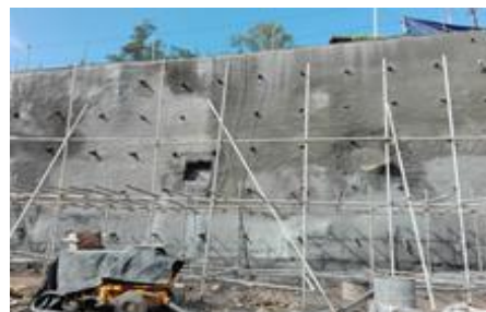
Rectification of failed slope at Diyathalawa Main Bus Stand
