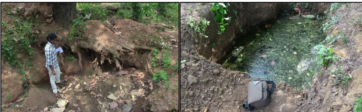
Figure 04: Identified hazardous locations.
