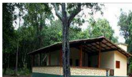
Figure 6.17: Renovated Manawila circuit bungalow in Wilpattu National Park
