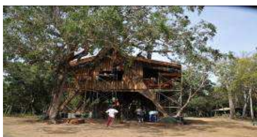
Figure 6.16: Sri Lanka Navy engaged in repair works at Kokmote circuit bungalow in Wilpattu National Park
