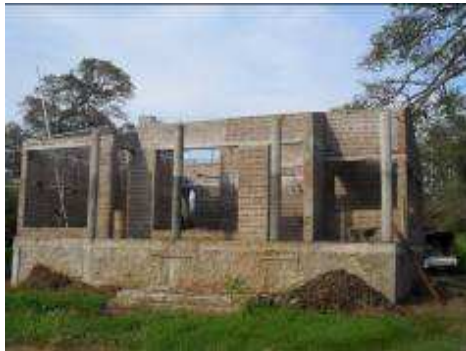
Figure 8.1: Construction of Ticketing Counter at Eluwankulama-Kalaoya Entrance
