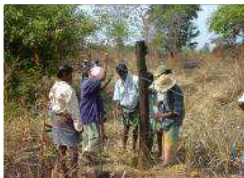
Figure 4.5: Fixing an electric fence
