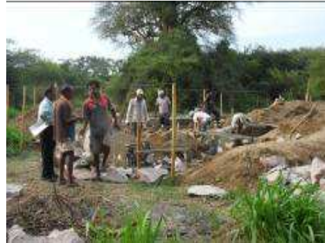
Figure 8.2: Construction of Staff Quarters at Kalaoya Entrance of Wilpattu National Park
