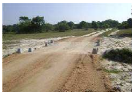
Figure 2.2: Rehabilitation of roads in Kumana National Park
