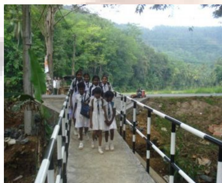
Construction of 02 Nos. of Foot Bridges at Meeriaama
