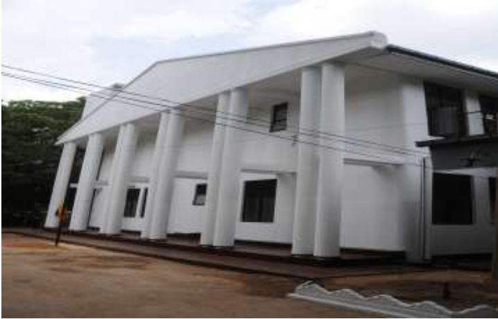
Vavuniya Civil Appeal High Court – Construction work is nearing completion.
