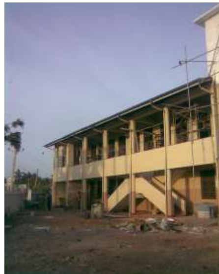
Mannar High Court Building
