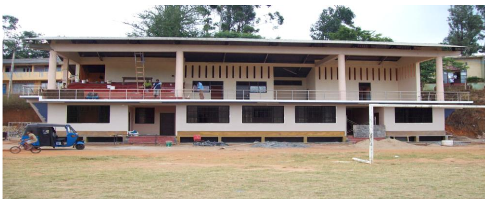
Construction of Ambagasdowa Sports
