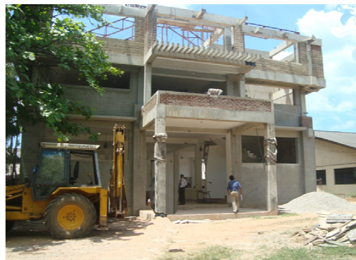
Construction Work is in progress
